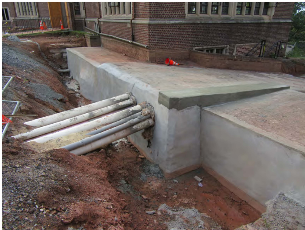
Underground Mechanical Tunnel Exposed After Concrete Repair of Roof Slab and new Shotcrete Walls.
