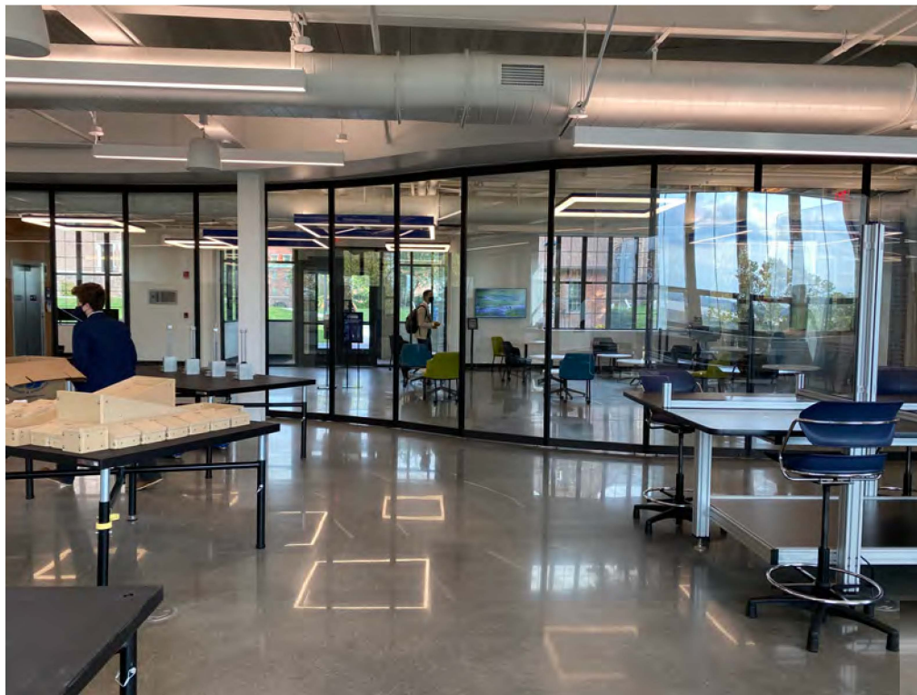
Curved Sliding Glass Partition Wall Separating the Lobby from the Engineering Lab, but can be opened to create a large event space.
